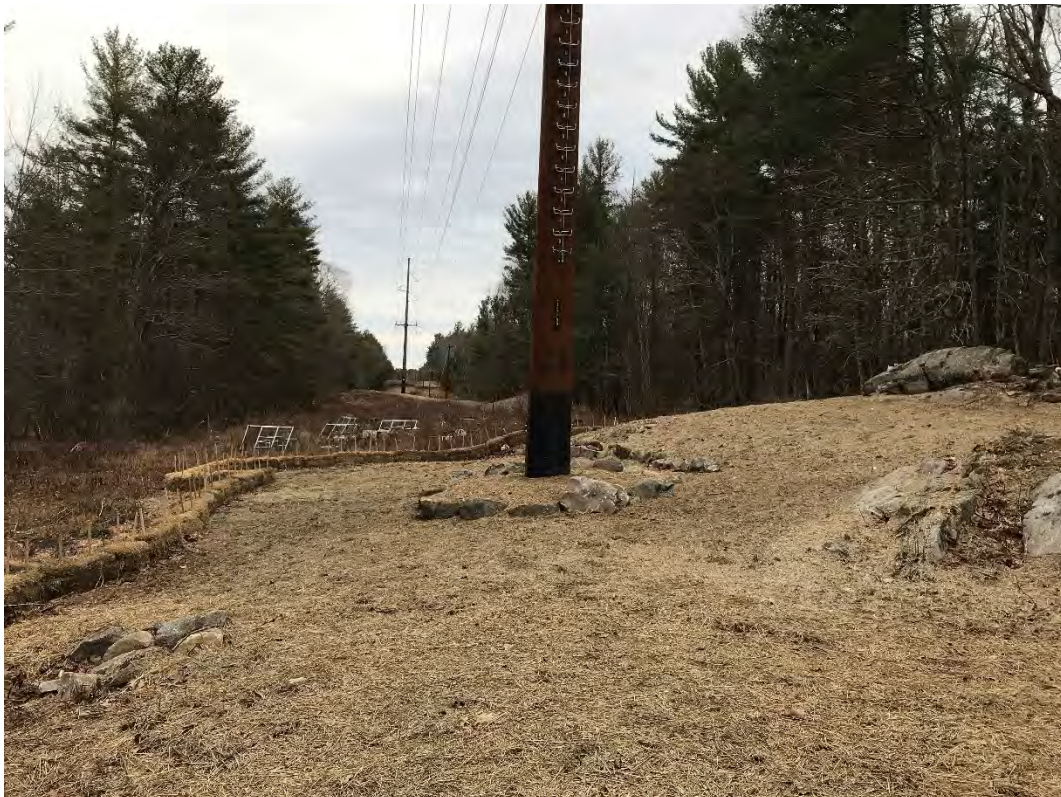
Fig 4: Str. 89 work area. Viewing southeast. (01-26-21)
