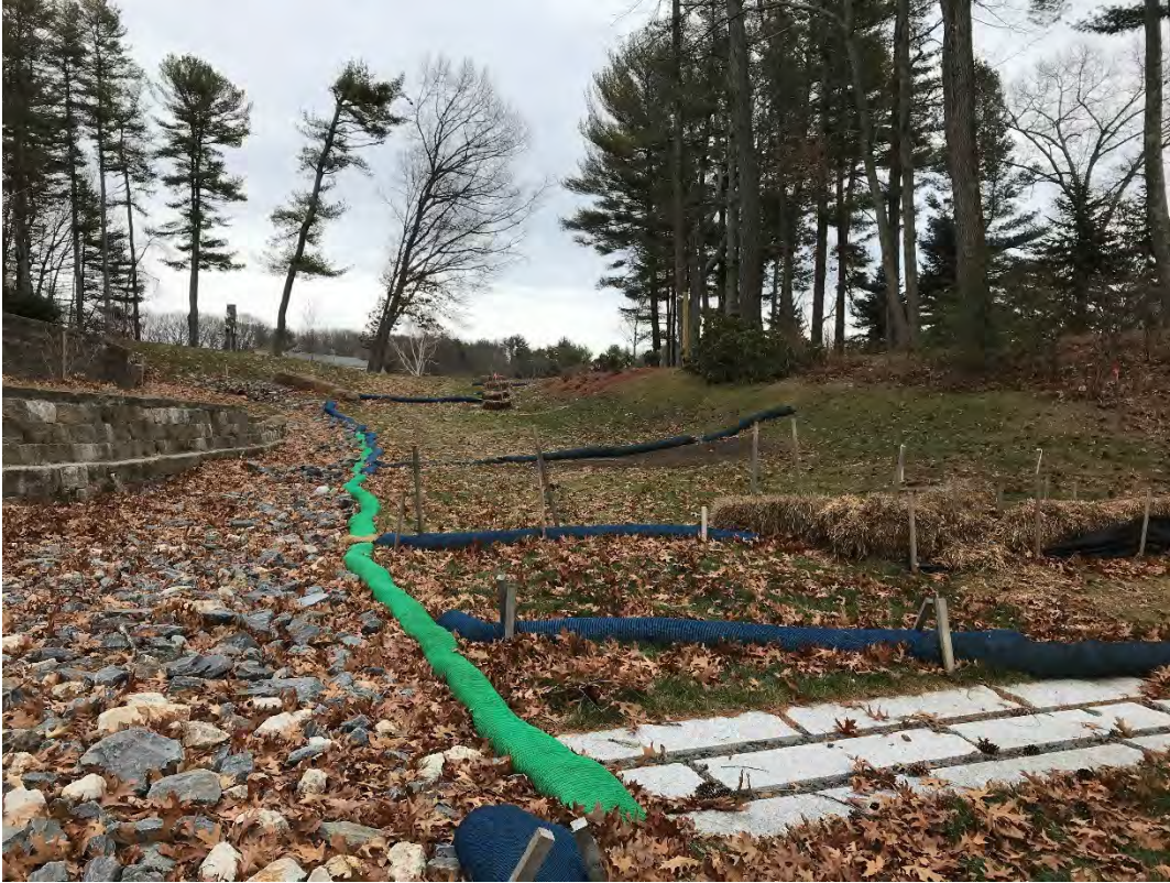
Fig 9: Slope above the manhole at Gundalow Landing/east side of the bay. Viewing east. (01-26-21)
