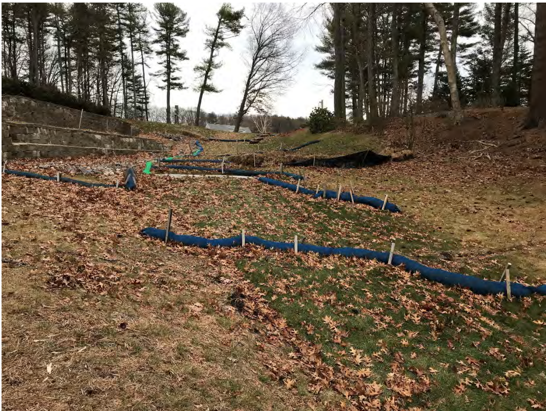
Fig 10: Slope below the manhole at Gundalow Landing/east side of the bay. Viewing east. (01-26-21)
