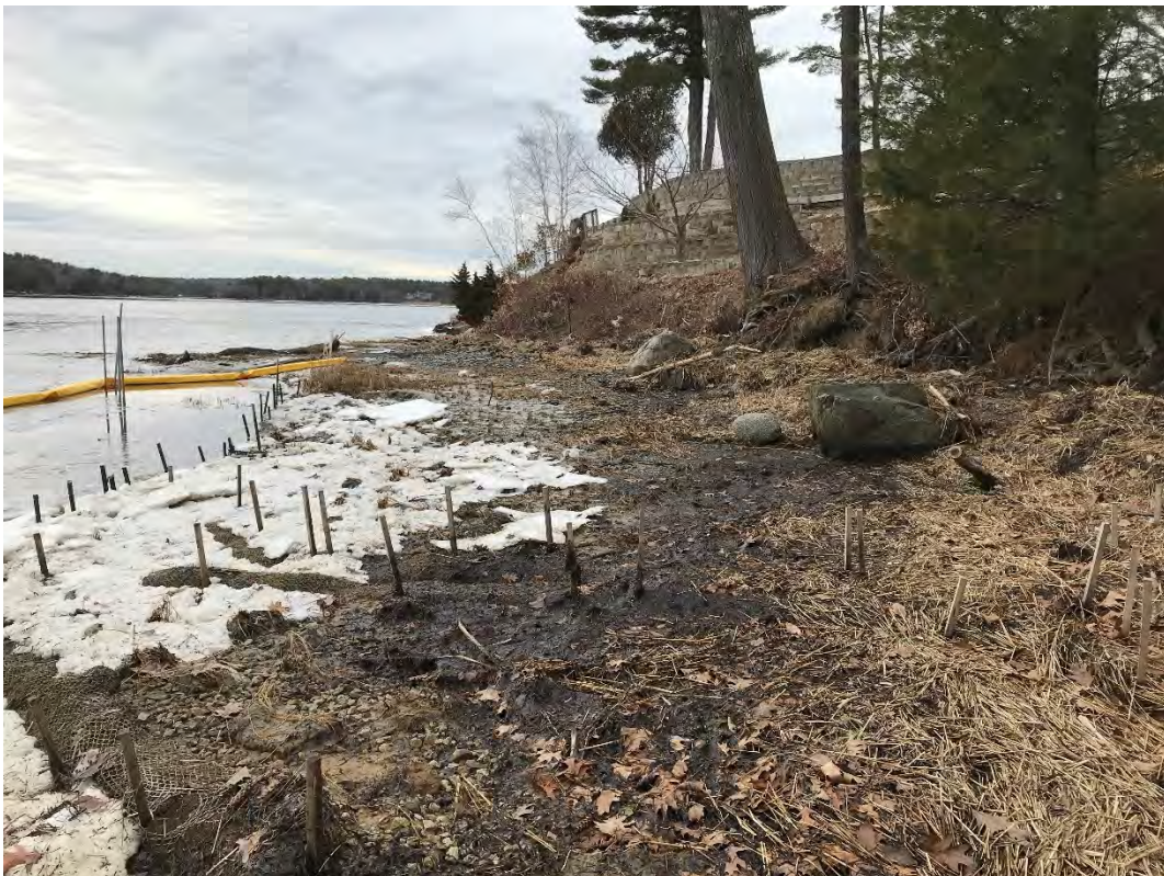
Fig 12: Salt marsh restoration at Gundalow Landing/east side of the bay. Viewing northwest. (01-26-21)
