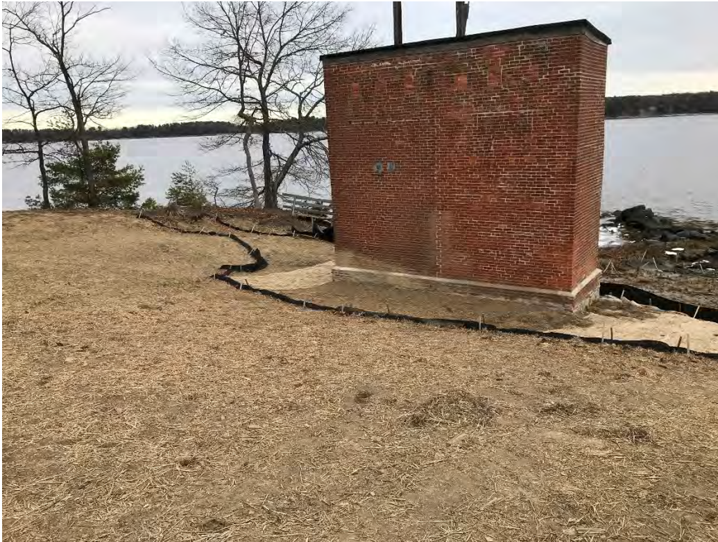
Fig 1: Slope leading down to cable house and salt marsh restoration at the Eversource property/west side of the bay. Viewing northeast. (01-26-21)
