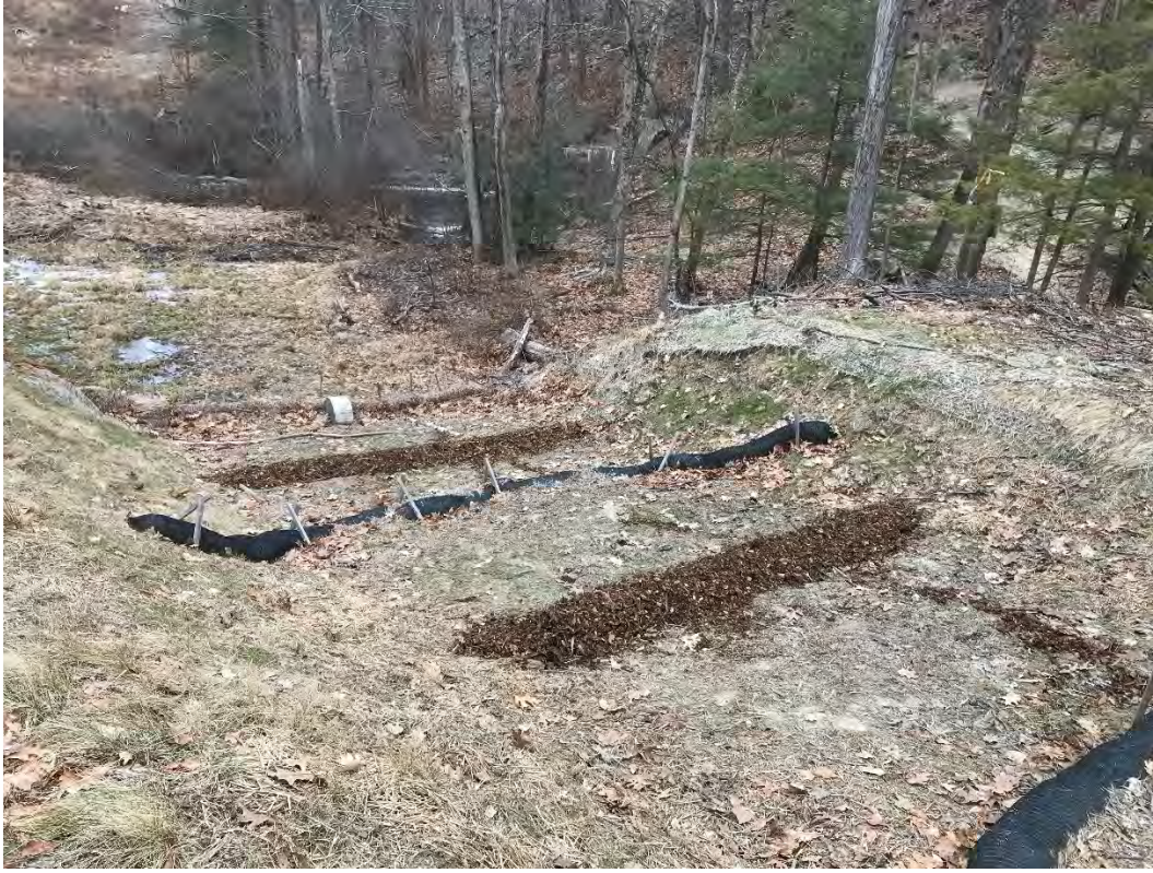
Fig 7: Lower portion of slope between Strs. 28 and 29. Viewing northeast. (01-26-21)
